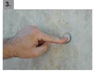
Close spacer tubes on both sides with sealing plug. In case of water tight binding sites, aditionnally use Fluppplug.
