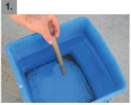
Immerse the BSS acoustic protection plugs into the water. (For fire protection application, use ANTIFLAME 2050 W!)
