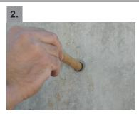
Insert the wet BSS acoustic protection plug into the binding site.
